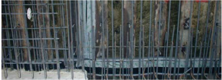
RGS intersecting installation
