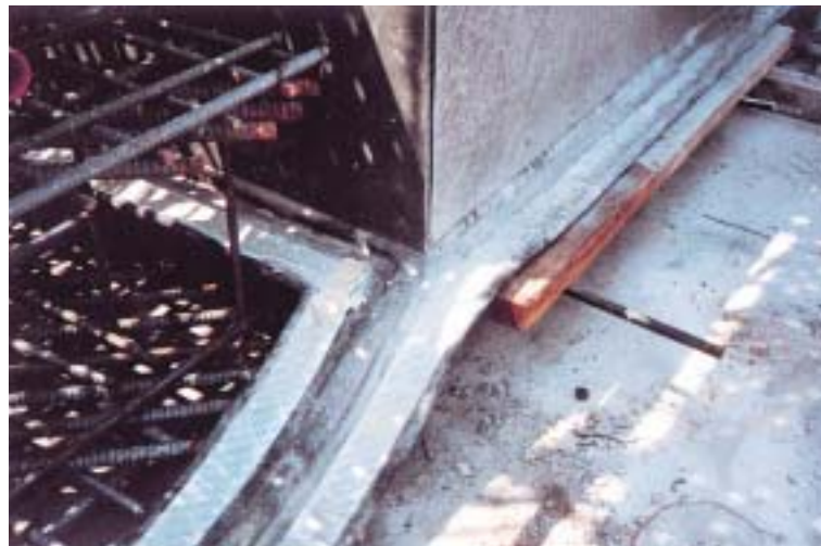
Condition of the waterstop after the primary concrete is poured.
