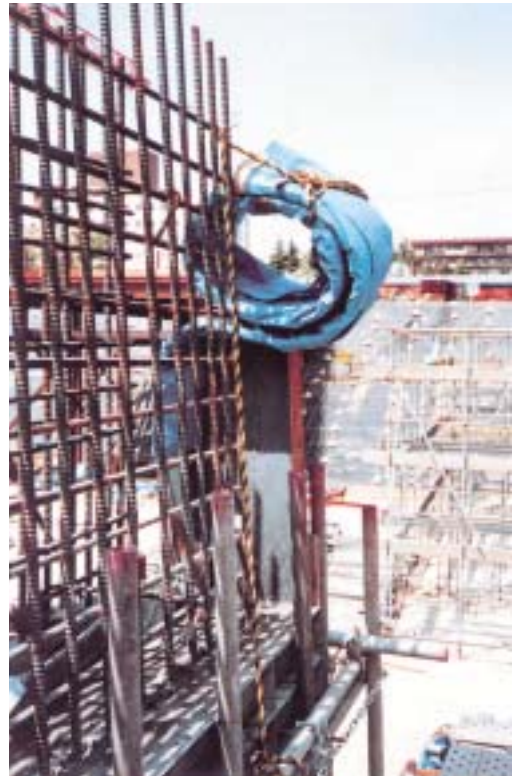
Edges of the waterstop covered with a protective sheet.
