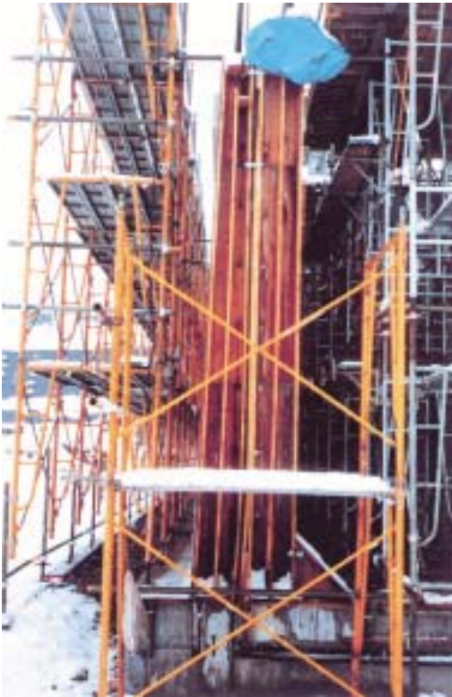
Waterstop firmly interposed waterstop between the forms.
